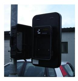
Open the sign and place the battery inside. The sign is now installed and ready for operation.
