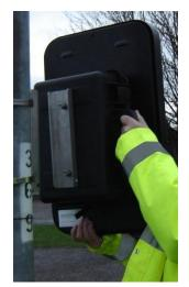
Carefully lift the sign on the bracket. The sign has two nuts that fit into the keyholes on the bracket. Once inside the keyhole, slide the sign down into the smaller part of the hole. When this is completed, the sign will be securely in place.
