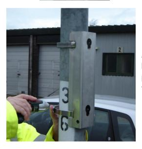
Make sure that the bracket is installed with the keyhole cut outs as shown facing outwards; the larger part of the keyhole towards the top with the smaller towards the bottom.
