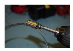
While pushing the fixing in this position, pick up the drill with the tamtorque bit and screw clockwise into the hole as shown on the left. This should then start to tighten around the post.
